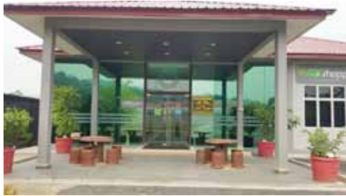
Plate 1. Front view of BBSHOPPE located at MARDI Headquarters, Serdang, Selangor
